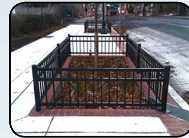
Micro-Bioretention, Towson, MD
