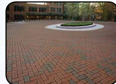
Permeable Pavement in Pedestrian Access Areas, Gott's Court, Annapolis, MD
